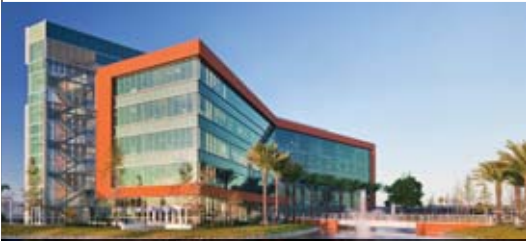
Headquarters of Adventist Health System in Altamonte Springs, Florida, United States. PHOTO: ADVENTIST HEALTH SYSTEM
